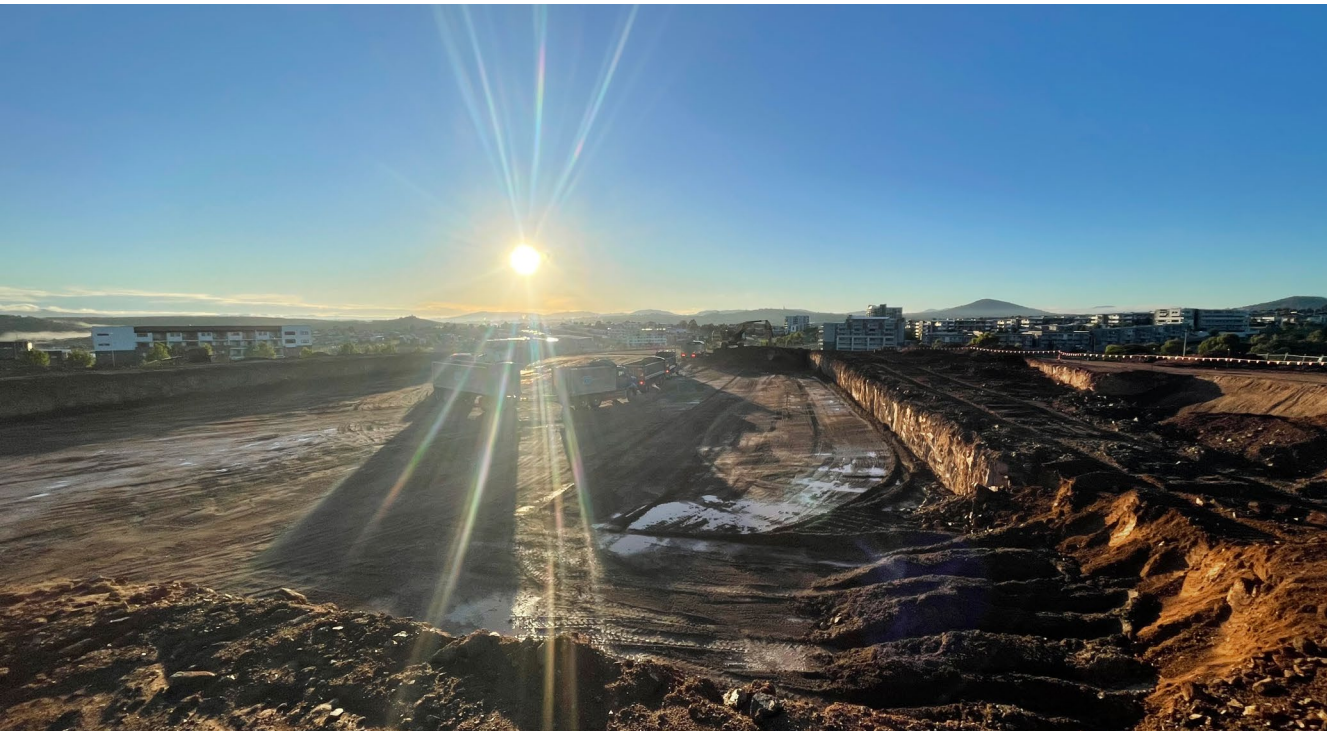
Stromlo Forest Anglican College site cut–February 2025
